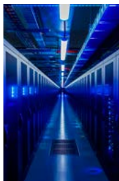
Electrostatic discharge flooring
